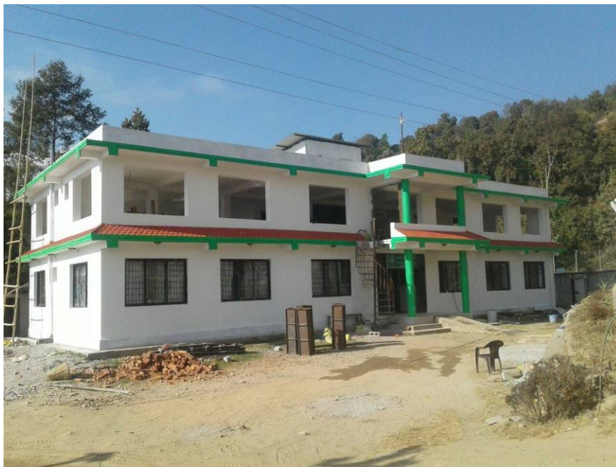
foto 9: De buitenkant is gereed (December 2016)
